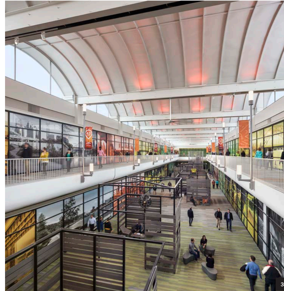
3. Nova Place Pittsburgh, PA, USA Urban mall converted to new office space
